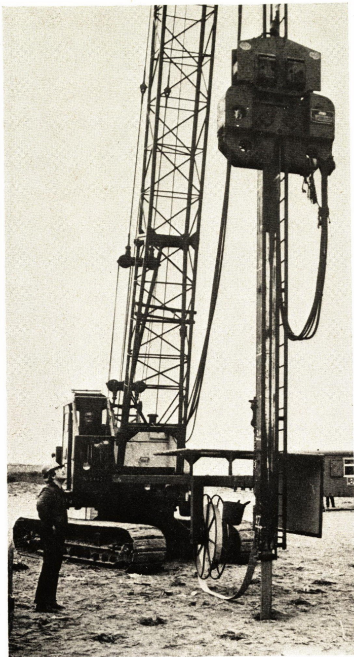
Fig. 6. Installation of Geodrain by means of a vibrating hammer. Contractor, Cofra (photo, Dienst Publieke Werken, Amsterdam)
